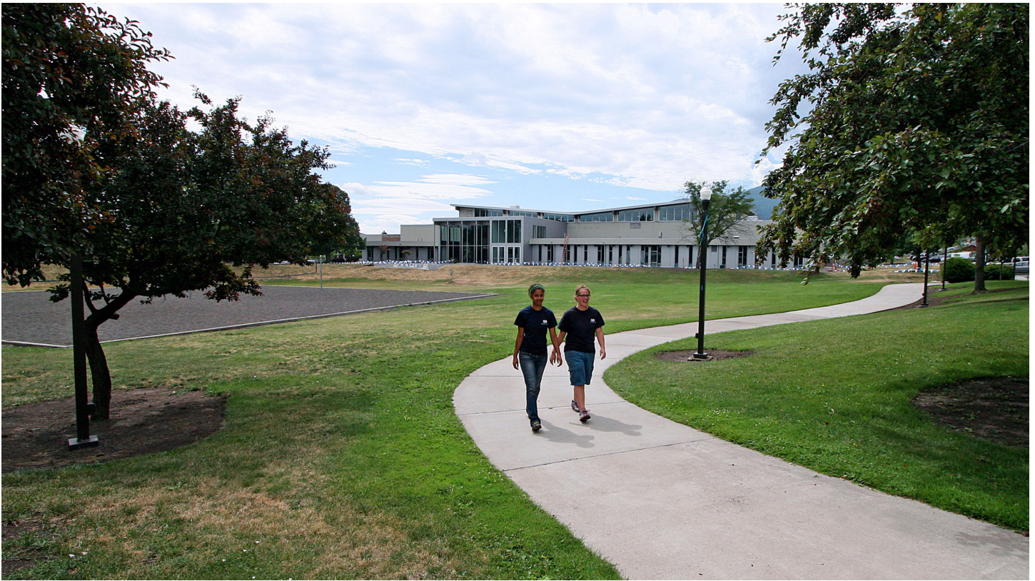
Quinn Coliseum renovation nearly complete fall of 2014. Fortis Construction, Inc. is the general contractor for the four capital construction projects which also included Pierce Library, Zabel Hall and Hoke Union Building.
